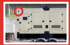
Attach the ViaCell-10 to a metallic surface to get notification of run status
